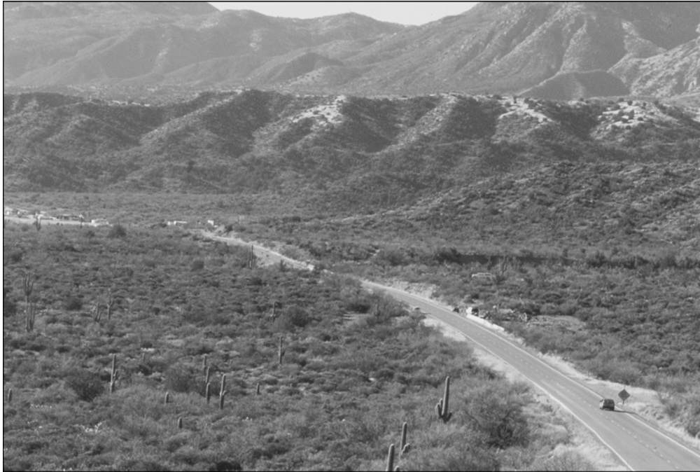
Figure 8. View south along SR 188 toward Slate Creek.
