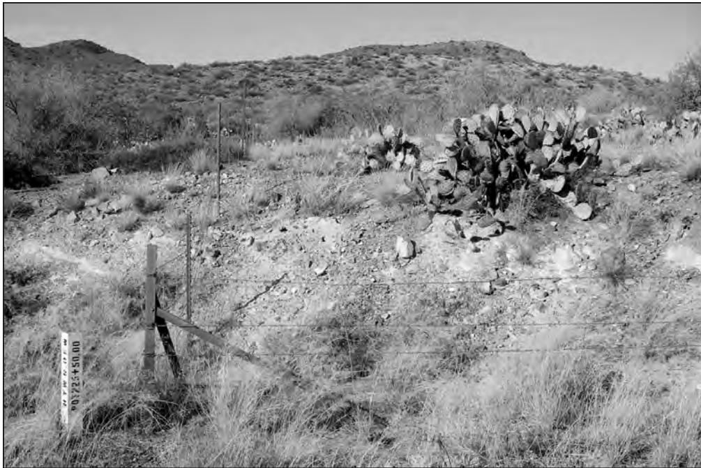
Figure 181. Roadcut 4 along Roadbed Segment 1, view west.
