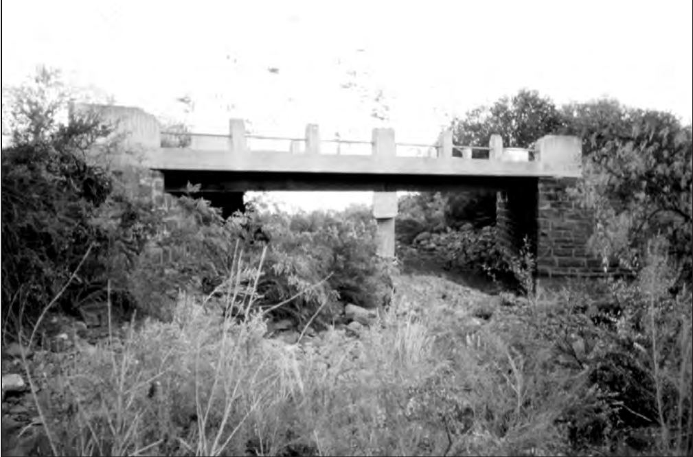
Figure 171. FH 9 bridge spanning Gold Creek.
