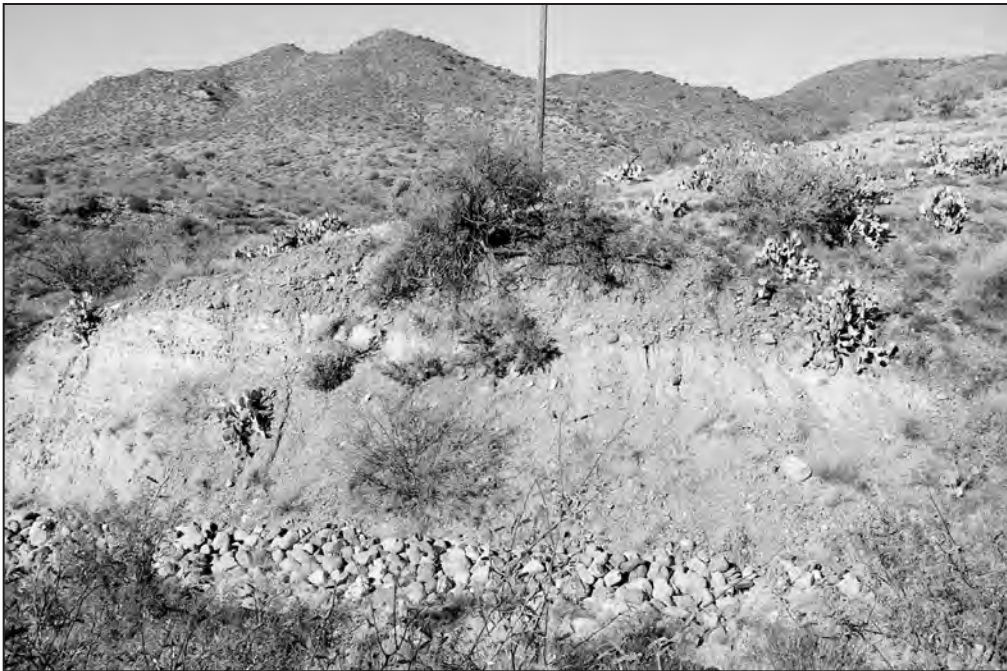
Figure 177. Roadcut 2 along Roadbed Segment 1, view west.
