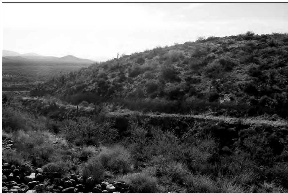
Figure 187. Roadbed Segment 4, viewed southeast from across the ravine.
