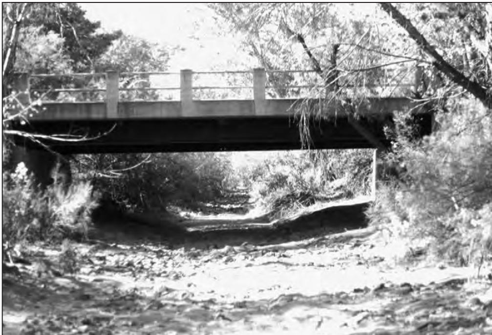
Figure 174. Hardt Creek Bridge near Jakes Corner.
