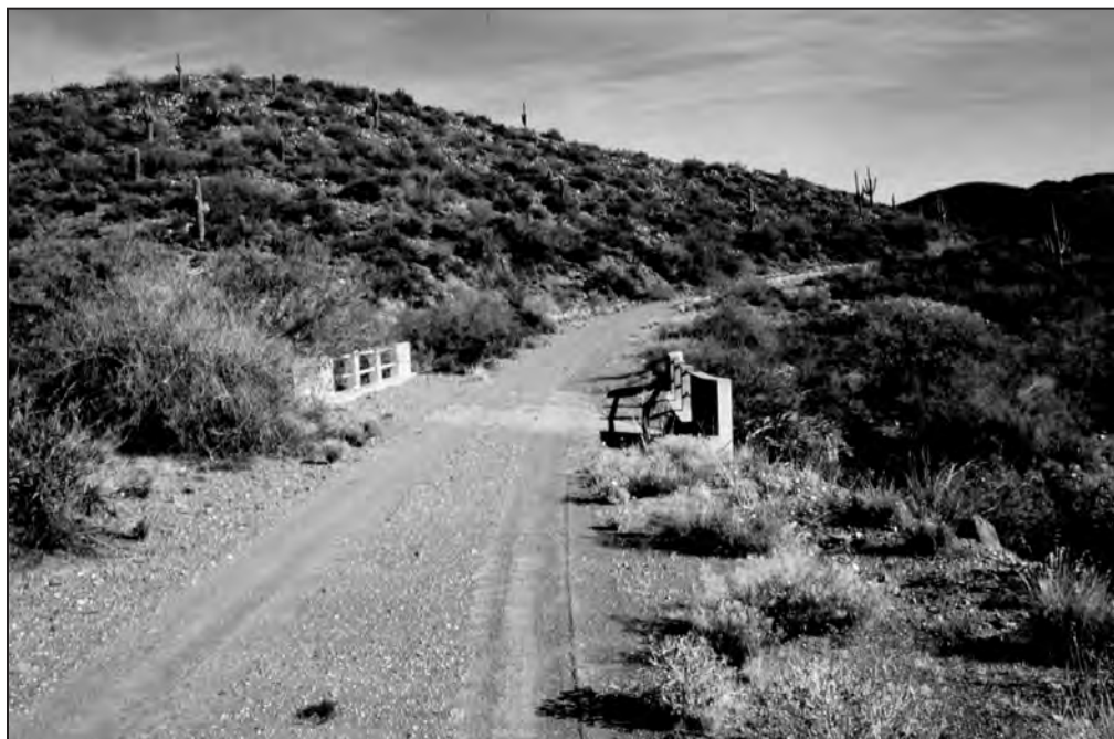
Figure 170. FH 9 roadbed over Reed Gulch Bridge, view north.
