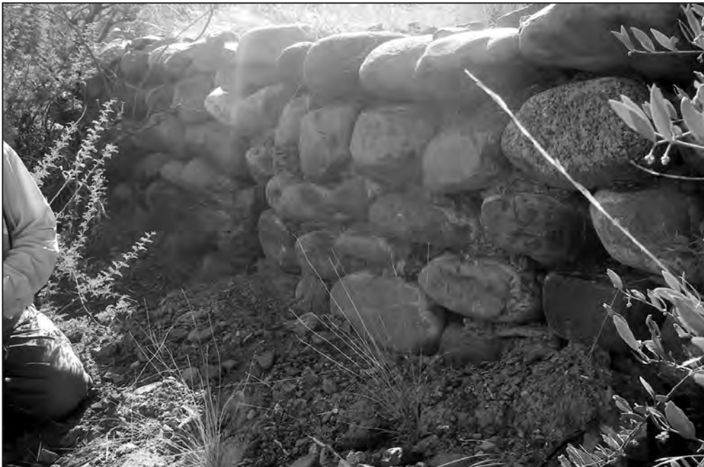
Figure 186. Detail photograph of dry-laid stone retaining wall, Roadbed Segment 3.
