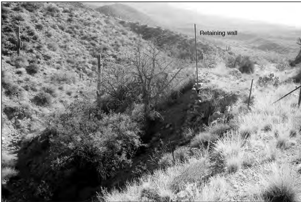
Figure 185. Retaining wall along Roadbed Segment 3.
