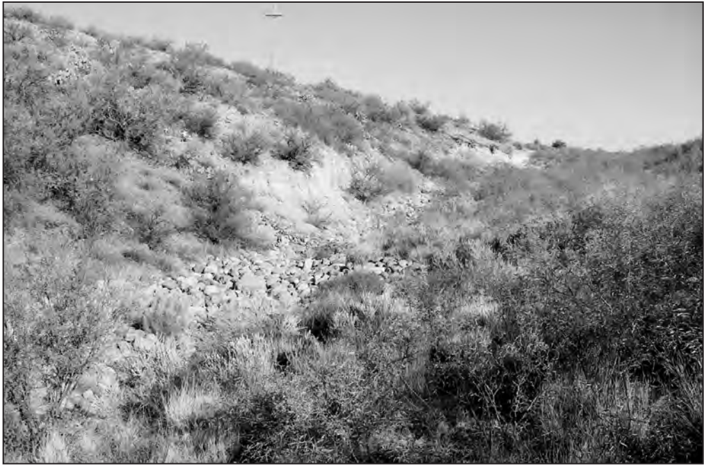
Figure 176. Roadbed Segment 1 along Roadcut 3, view north.
