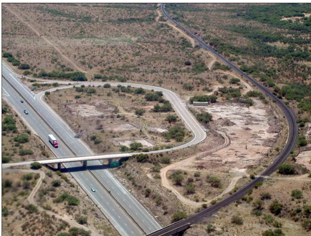
Figure 53. Aerial overview of Locus C (left center, enclosed between roads) after excavation; view to the southeast.
