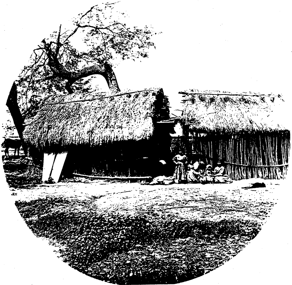
Figure 4.1. Indian jacales (brush houses) at Sunny Slope Vineyard near San Gabriel, perhaps photographed during the 1850s or 1860s (courtesy of the Sunny Slope Water Company).
