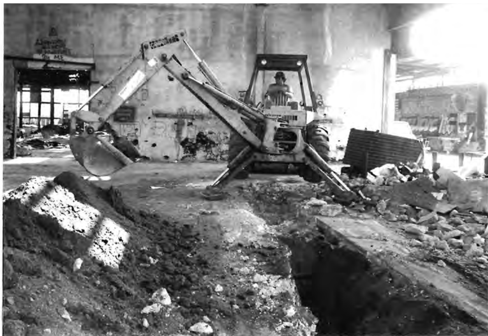
Figure 36. Photograph of Case backhoe excavating trench inside the Associated Pacific Building.
