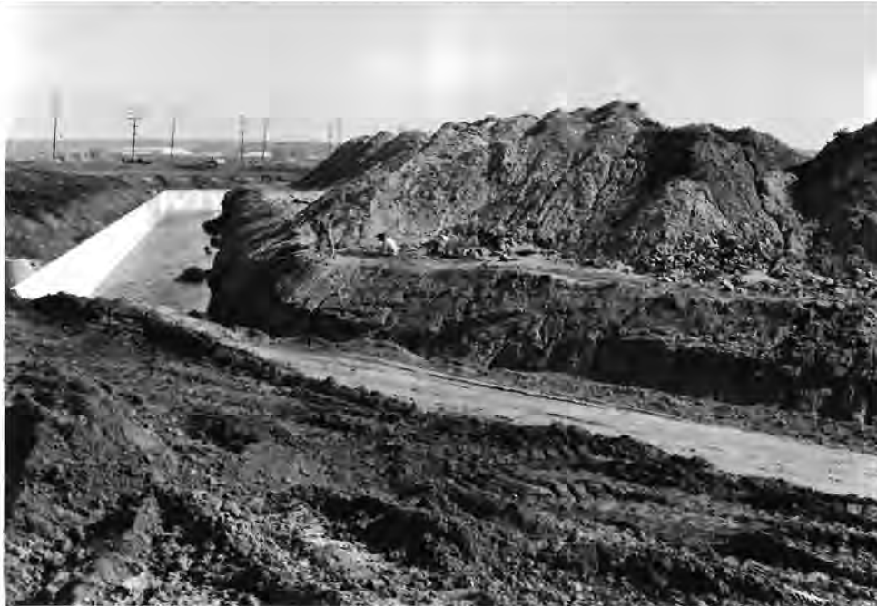
Figure 33. View of eastern excavation unit, looking south. Note: This excavation area is now within Basin F of the Marina del Rey Harbor (Photograph courtesy of Keith Johnson).
