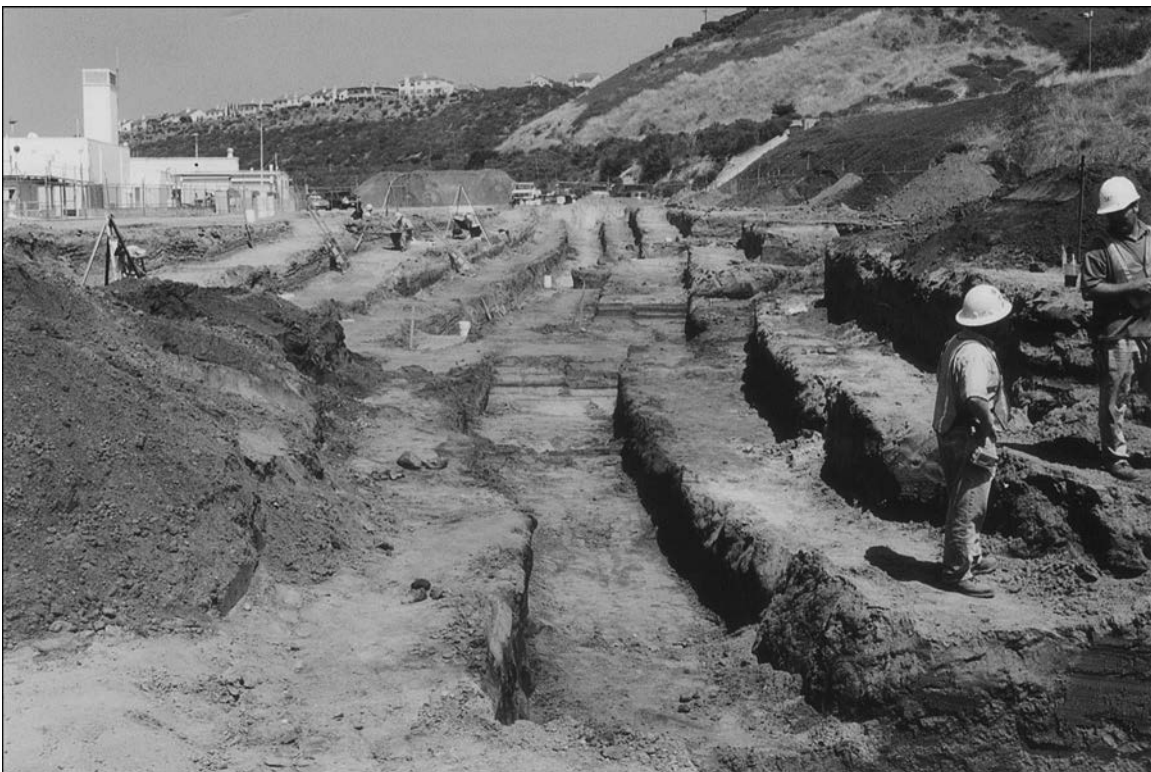
Figure 86. Photograph showing the stepped trenching operation, LAN-193, view to the east.
