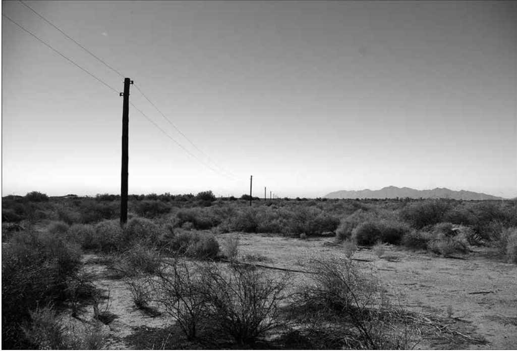
Figure 258. Original utility poles and power lines.
