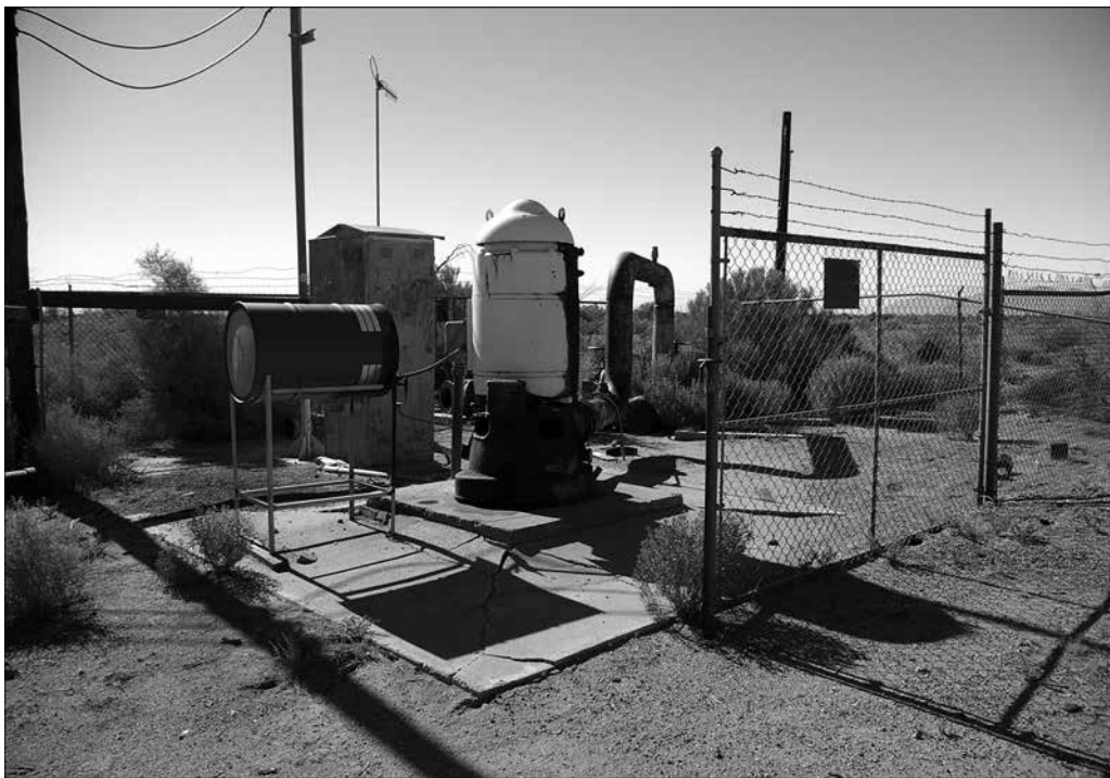
Figure 257. Well site, view to the southeast.
